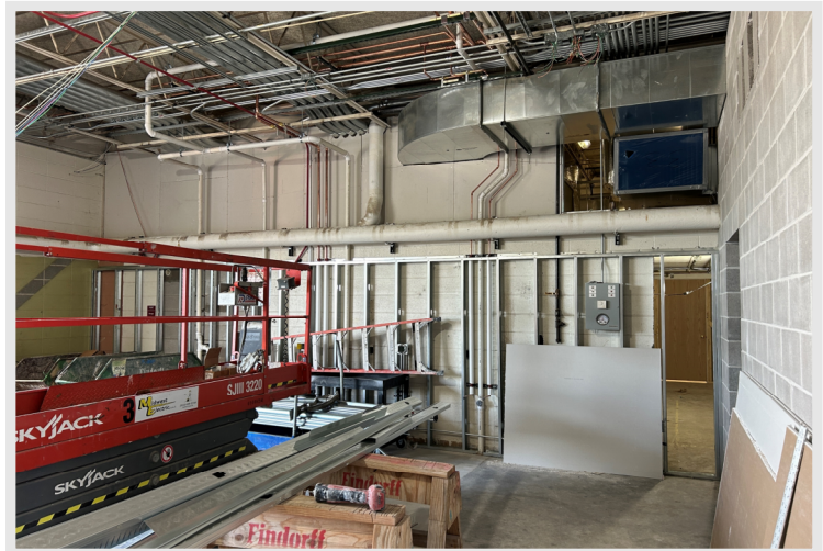
Findorff carpentry crews, alongside MEP crews, have built up stud walls in the Test Kitchen/Head House areas ahead of new drywall finishes.
